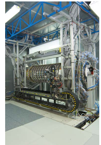
Low operating temperature anti-static, raised access flooring system - ATLAS Detector, Large Hadron Collider Project.
