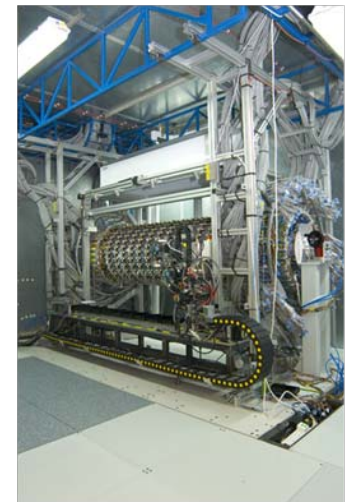
Low operating temperature anti-static, raised access flooring system - ATLAS Detector, Large Hadron Collider Project.
